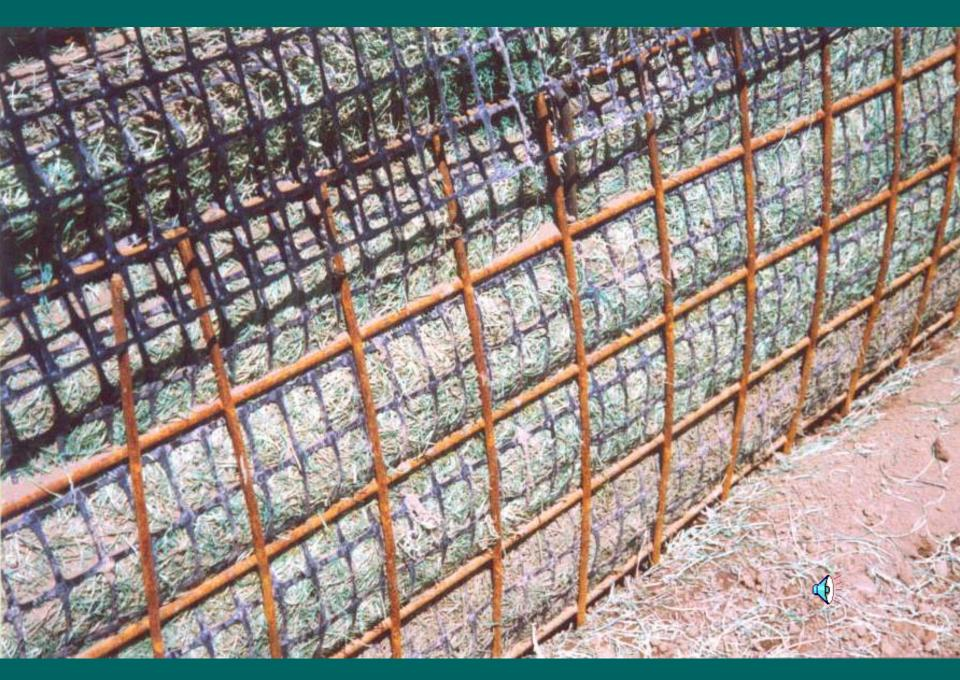
Seeded Erosion Control Material/Bidirectional Geogrid/Welded Wire Mesh
