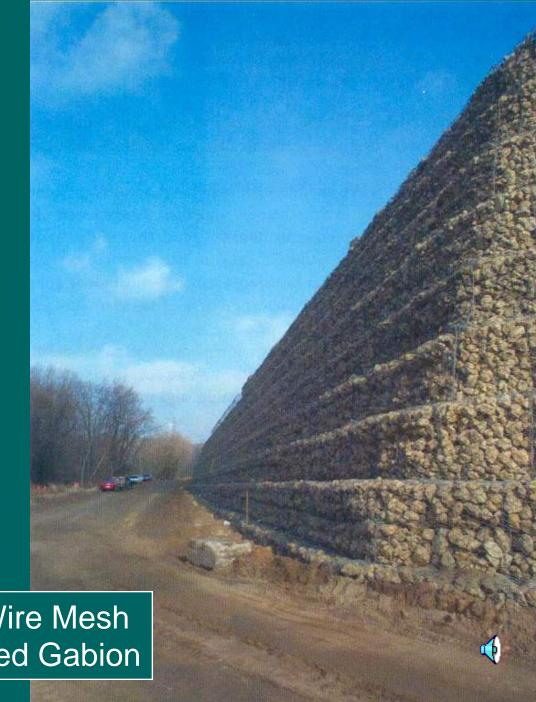
Welded Wire Mesh Stone Filled Gabion
