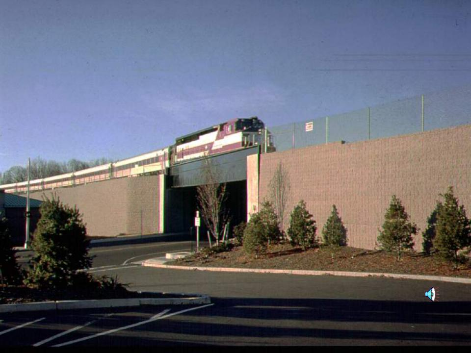
Photo 1. Segmental retaining wall (SRW) components of a completed bridge abutment.
