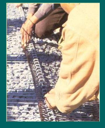
Tensar's SierraScape™ Using Welded Wire L-Bracket
